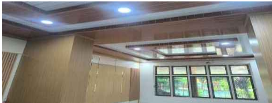
Gambar 3.5 Rehab Gedung SMA Lab School
